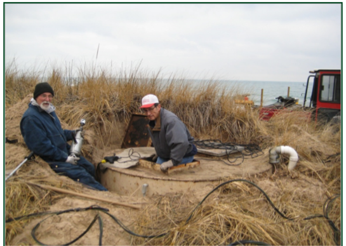
Mark Bapst and Irv Call boring through the Caisson for the power line shown in the foreground (Note: The Caisson is a round silo like steel vessel buried in the ground. Inside it is about 7 feet high and about 7 feet in diameter.)
