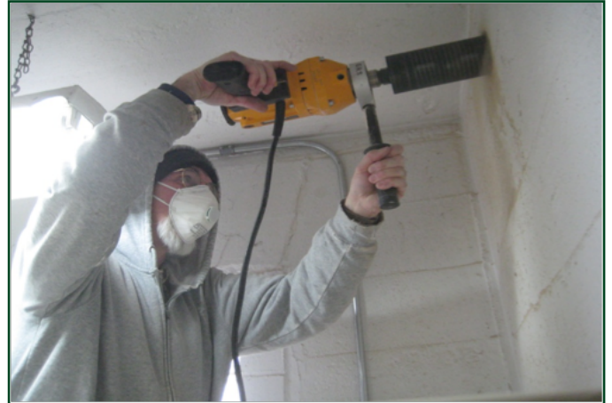
Mark Bapst boring through 10.5 inches of concrete
