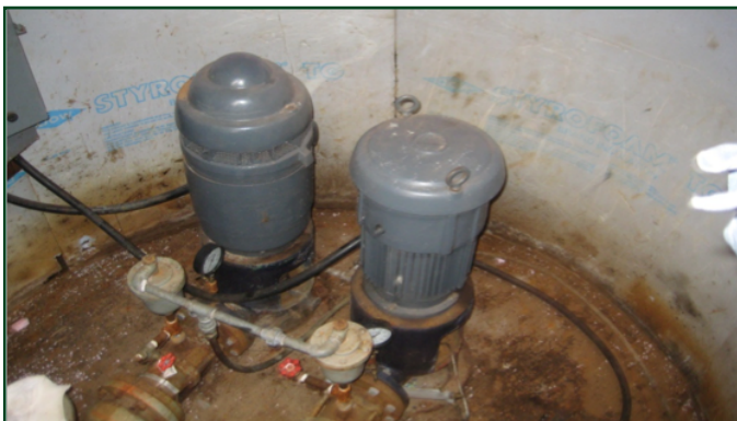
Inside the caisson are two pumps which pump "lake" water to the tank at the Maintenance Building. Shown are vertical standing motors which drive the pumps 8 feet below the floor.
