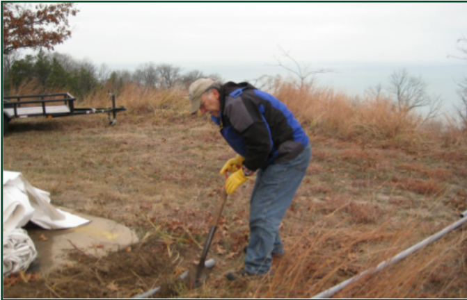
Ivan Chermel burying conduit running to the Maintenance Building
