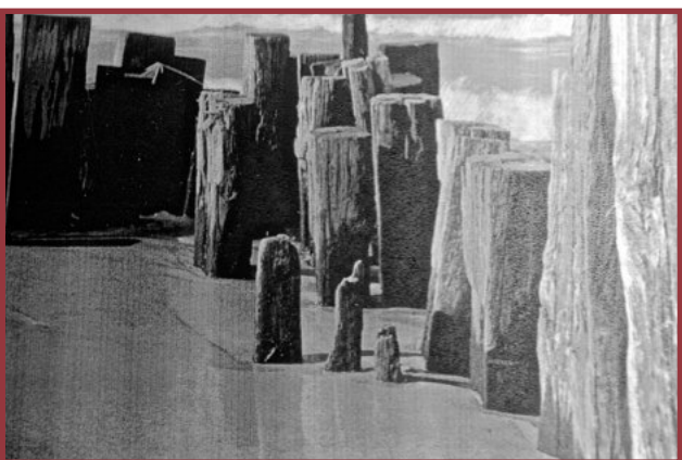
Vertical railroad ties installed as a breakwater after the 1929 storm were exposed after the 1951 storm.
