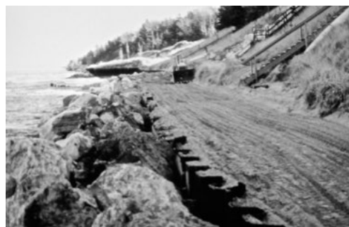
In front of Shore Dr homes: Nearest the water: riprap boulders; next, first row of installed steel pilings with sand filled-in behind; then, leveling sand in preparation to install a higher, second steel and wood wall along the dune bluffs.
