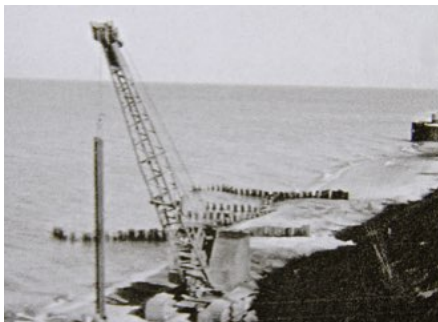
Pilings being installed in '71 in front of Roberts' home. Wooden pilings installed in '51 in front of Col. Melton's home reappeared in '71.
