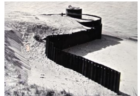
Steel pilings with back-filled sand protect Town Pumps
