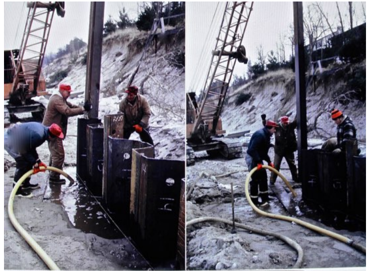
Bob Greer driving steel pilings down 15" and exposed about 4'. Most home- owners installed steel walls which connected to form a solid front. They then backfilled the dune from the lake.
