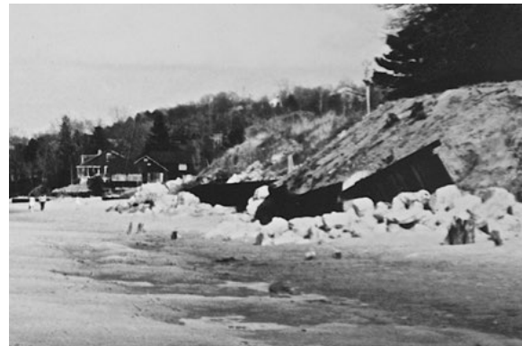
The '51 pilings in front of Beach Dr could not withstand the invasions of '71 and '72..
