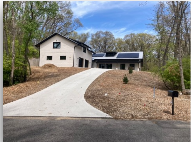
18 Panel 9 KW Solar System on south facing roof.
